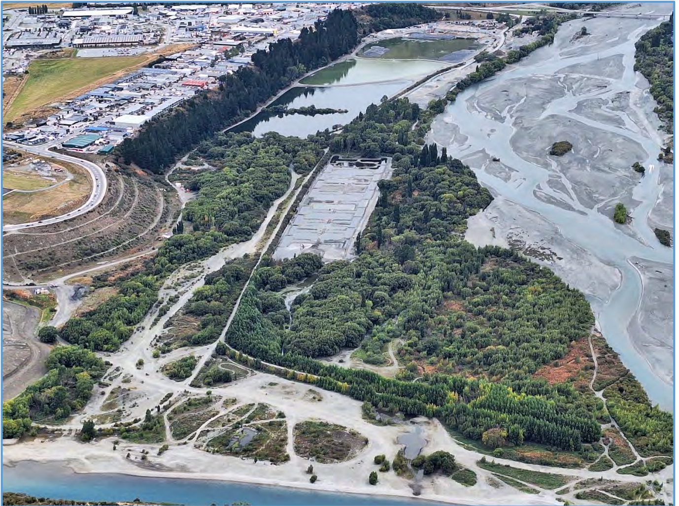
Figure 3: Image of the Property taken from the Remarkables by ORC Enforcement Officer 4 March 2024. Showing the extent of the ponding within the Disposal Field and outside the Disposal Field boundary.
