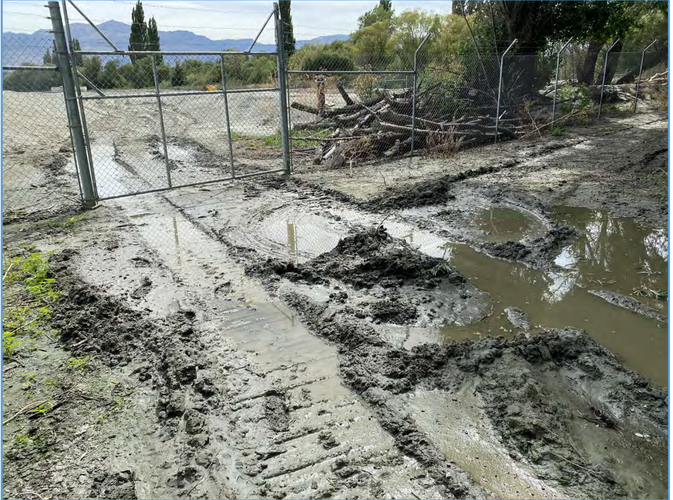
Figure 21: The SSE corner (which had breached previously on 27 December 2023) was now saturated with wastewater under and around the Disposal Field gate. There was a visible flow path from the Disposal Field towards the gate. There were puddles of liquid present that hadn't been there the previous day. There were also fresh heavy vehicle track marks observed.
