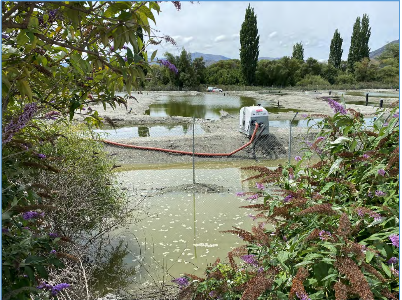
Figure 16: A significant breach and ponding of wastewater extended approximately 100 metres by 3 metres wide outside the consented Disposal Field boundary, between the boundary and the public cycle path.
