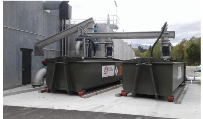
Figure 6: Sludge bins and loading conveyors
