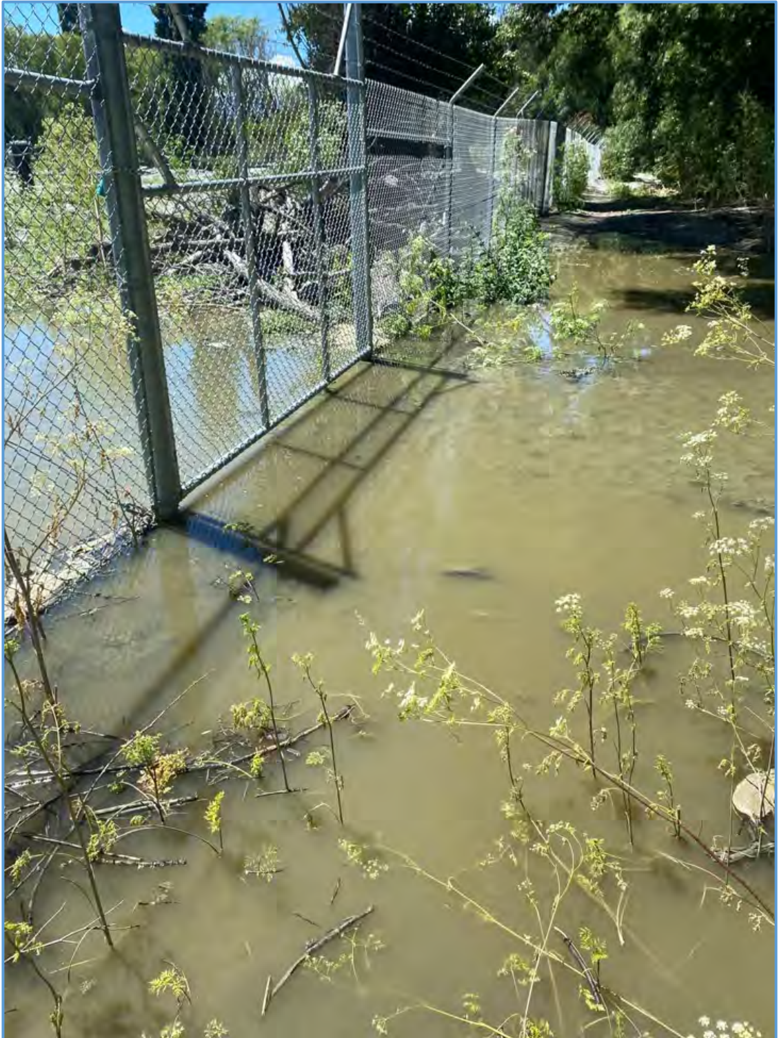
Figure 5: A substantial flow discharging from the bottom SSE corner discharging beyond the consented Disposal Field boundary.
